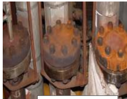
Inspection Of Top End
