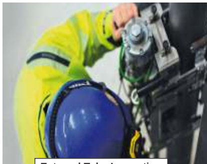
External Tube Inspection (LEO-Scan)
